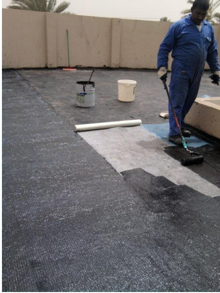
Applying a second layer of Leyco Plast over the Leyco Mesh
