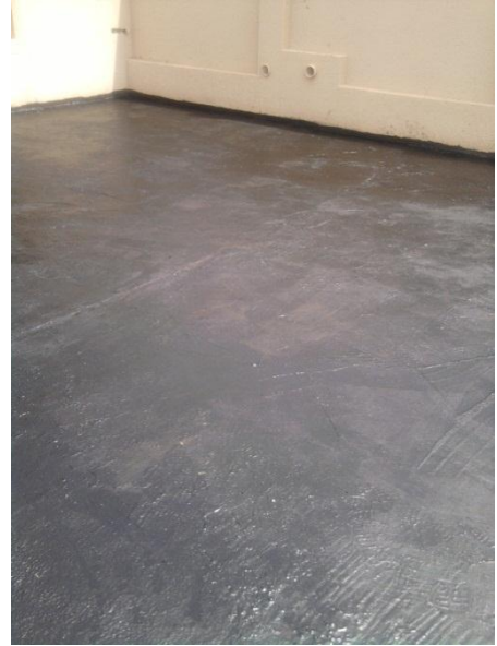
Surface is ready for the Leyco Tiles
