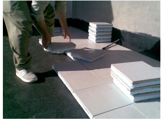
Placing the Leyco Tiles – Easy & Fast application
